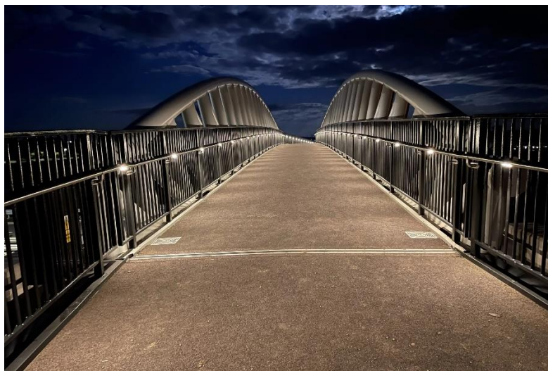
Broomhall Way Footbridge Southern Link Road A4440, Worcester
