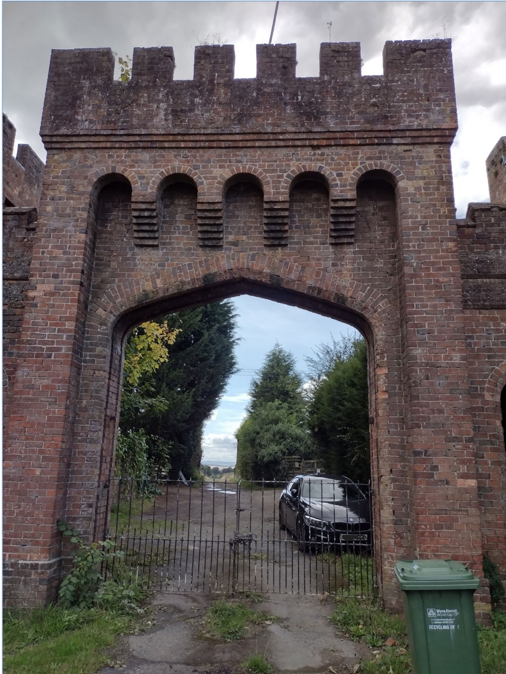
Photo 1: Listed Gateway, from Wolverhampton Road, looking south-west in the direction of the Appeal Site
