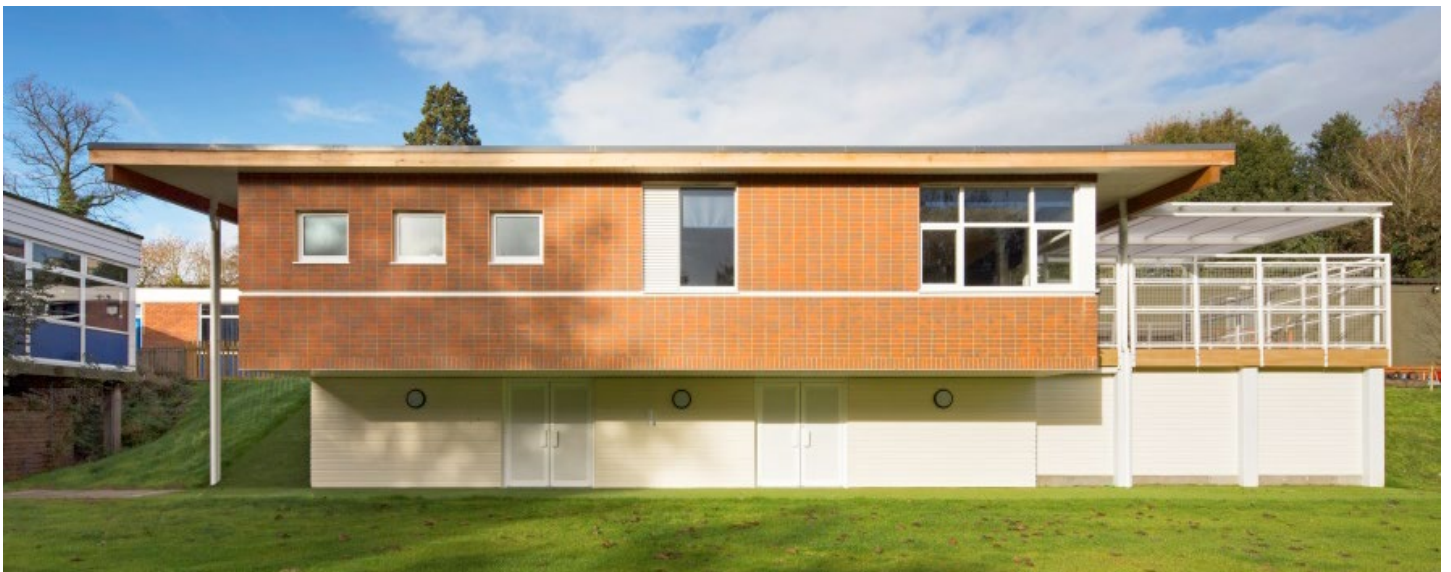
Rigby Hall School - Extension
