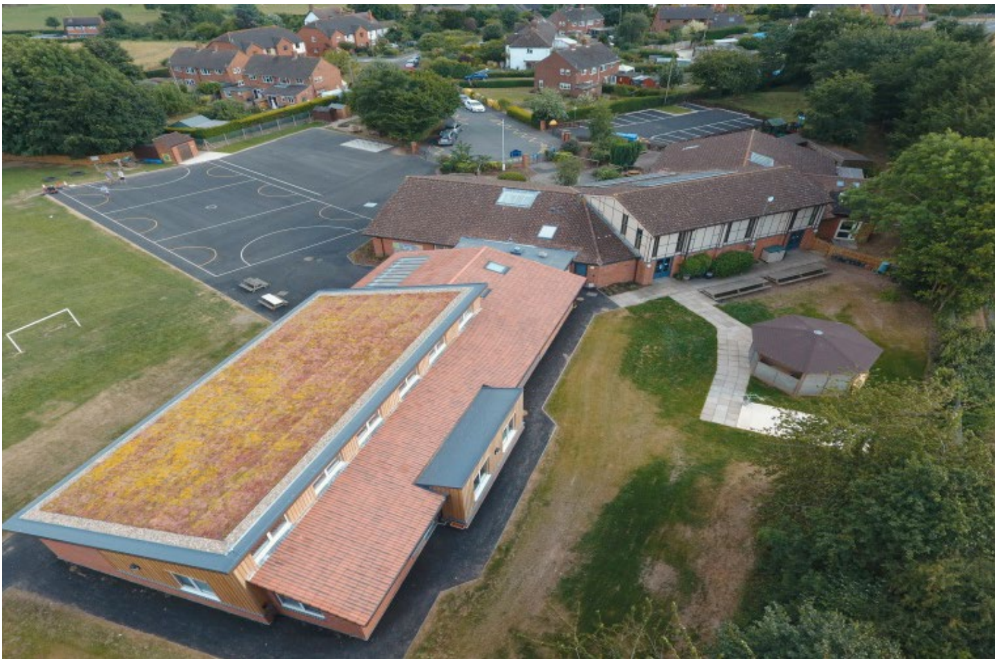
Leigh & Bransford Primary School - Extension
