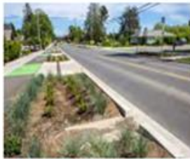
Low-level rainwater garden
